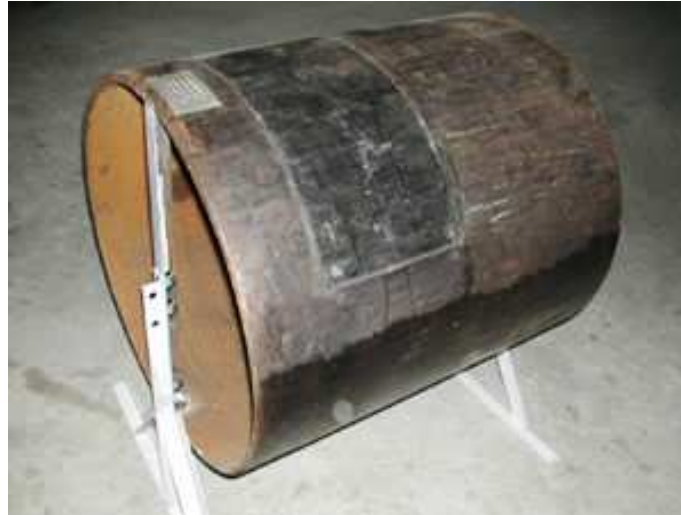
Oil Pipeline Inspection
